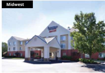
Fairfield Inn & Suites
