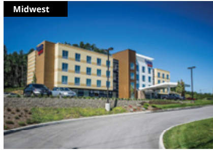
Fairfield Inn & Suites
