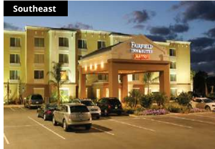
Fairfield Inn & Suites
