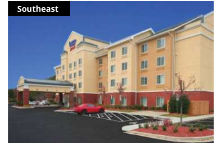
Fairfield Inn & Suites
