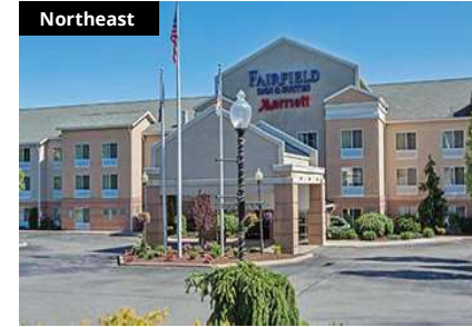
Fairfield Inn & Suites
