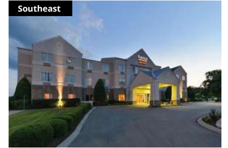
Fairfield Inn & Suites
