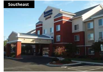
Fairfield Inn & Suites
