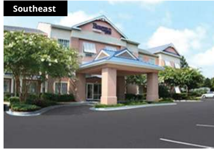
Fairfield Inn & Suites
