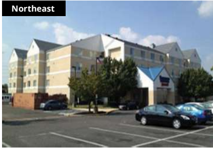
Fairfield Inn & Suites
