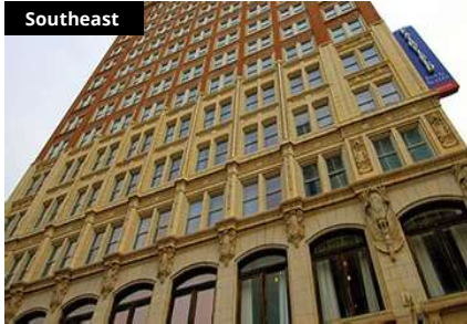
Fairfield Inn & Suites
