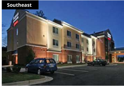
Fairfield Inn & Suites
