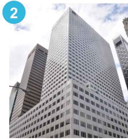
666 Fifth Avenue (office) $1,286,083,000
